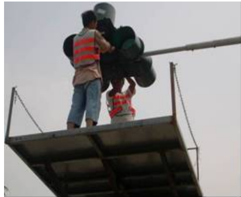
LED 燈面更換作業
